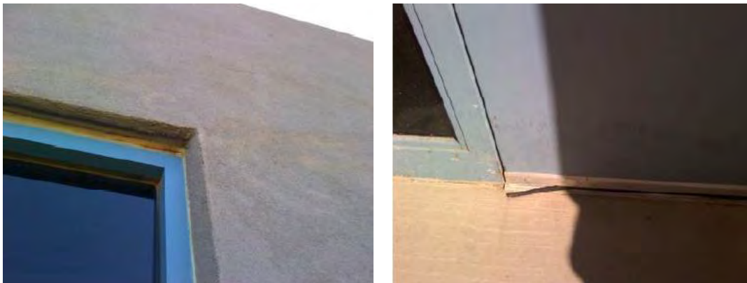
Figure 20: Flaws in building envelope at La Familia Medical Center
