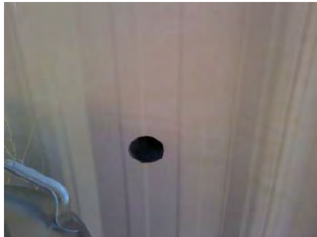
Figure 40: Building Envelope Gaps at the Santa Fe Regional Airport
