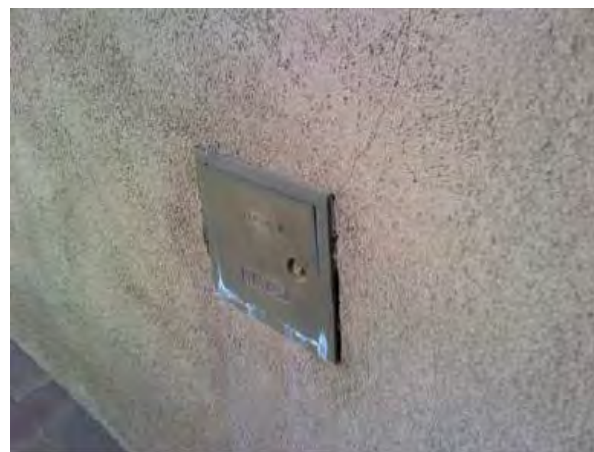
Figure 35: Building Envelope Gaps at SFCC
