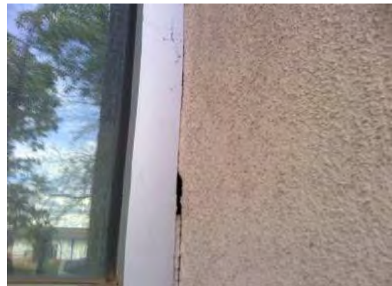
Figure 44: Gaps in Building Envelope at Siler Complex Building C
