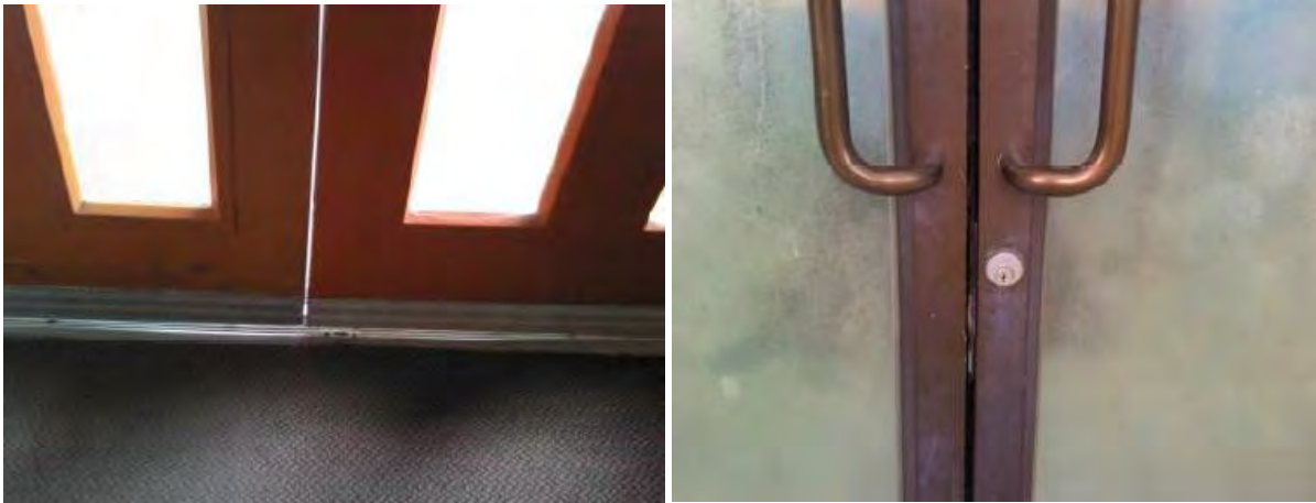
Figure 7: Gaps in building envelope at Alto Complex
