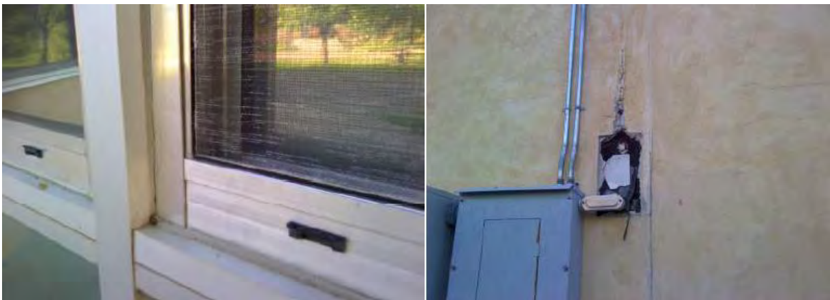
Figure 47: Additional Gaps in Building Envelope at Siringo Complex Warehouse
